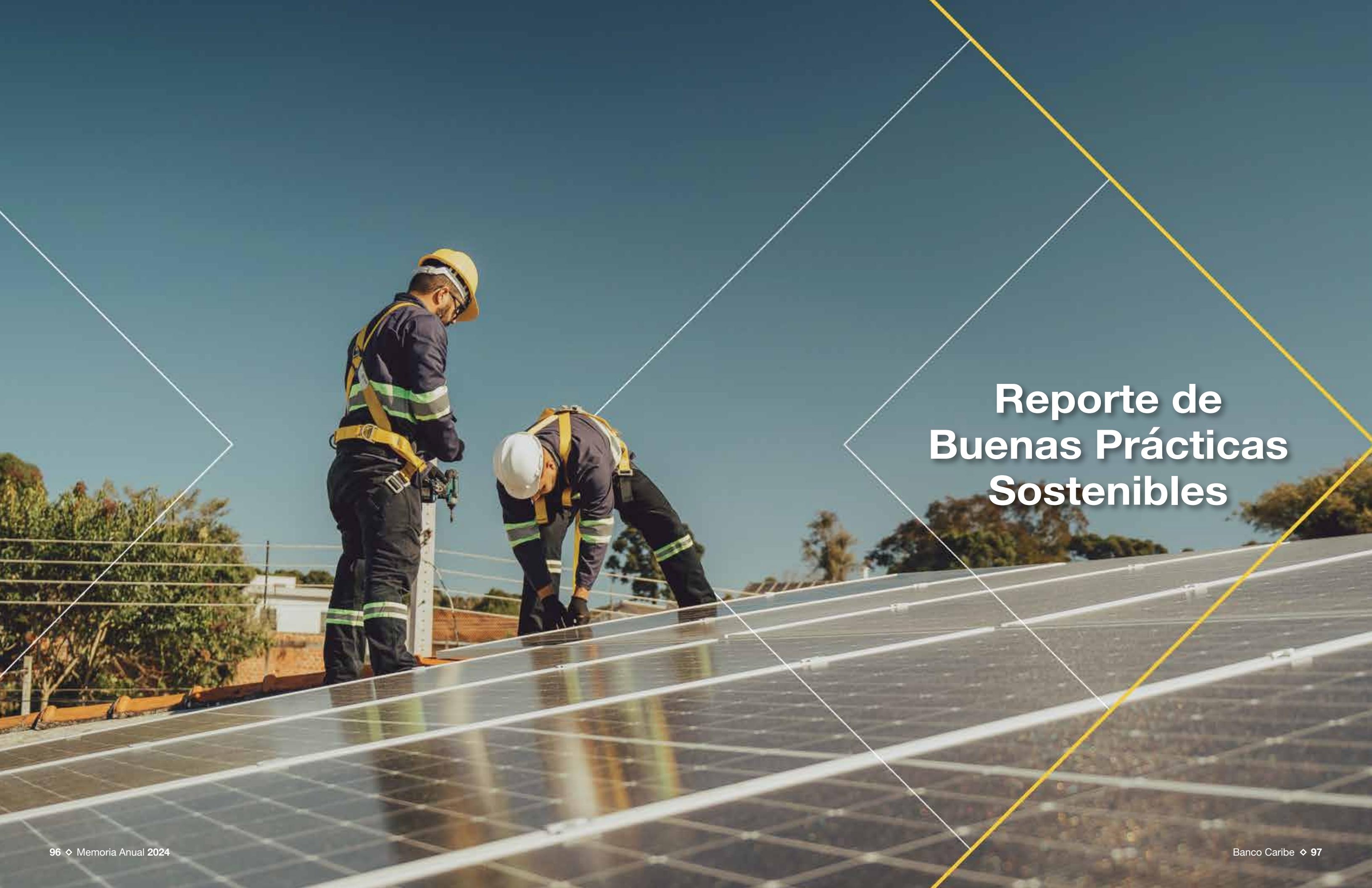
A photograph showing two workers in safety gear (hard hats and high-visibility vests) installing solar panels on a roof. One worker is standing and holding a panel, while the other is kneeling and working on the mounting structure. The roof is covered with many solar panels, and the background shows a clear sky and some trees.
